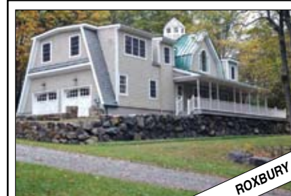
Quality New Construction. 4 Bedrooms. Fireplace. 4± Acres. Great Location. EXCLUSIVE $1.295.000.
